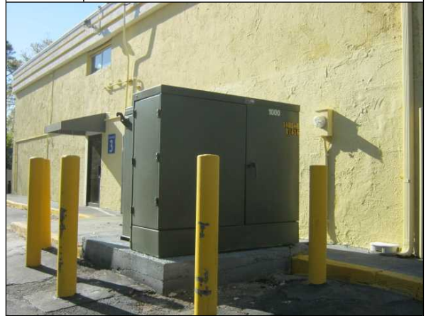
36. Pad mounted transformer.
