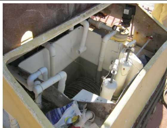
30. Swimming pool filter equipment.
