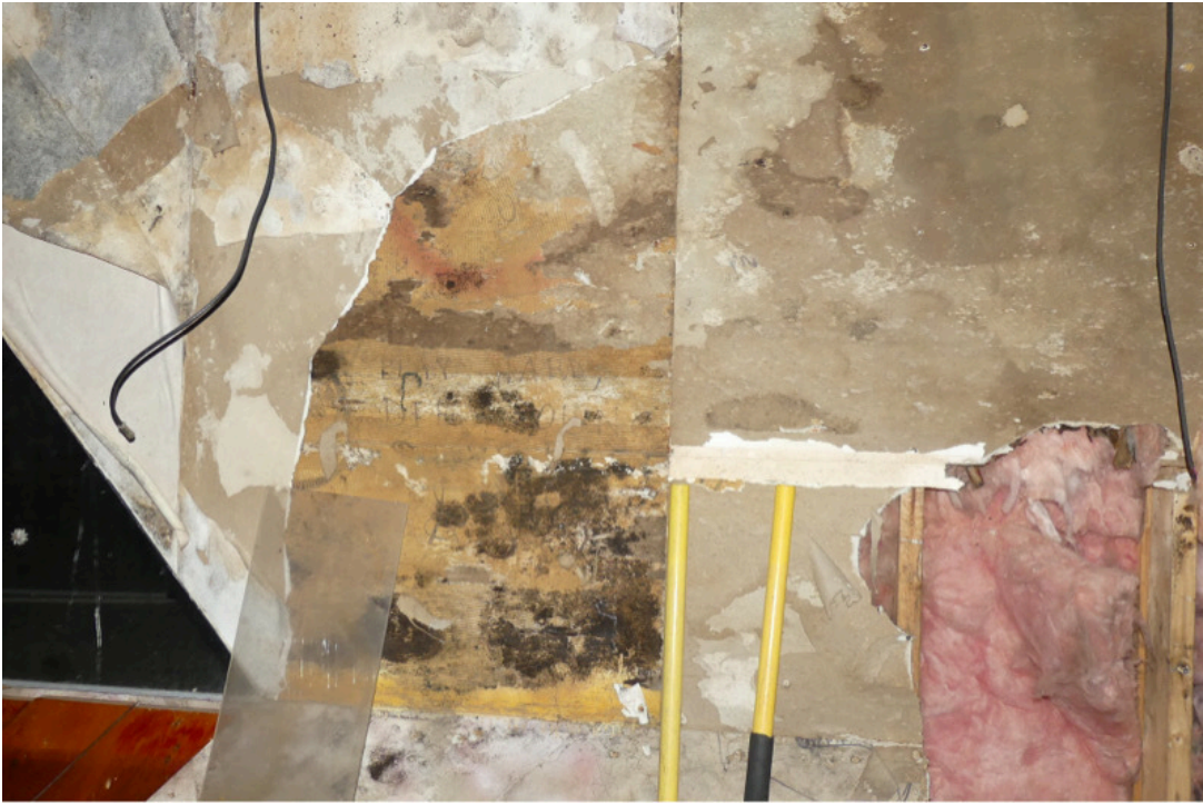
51. Mold and moisture in the former bar area
