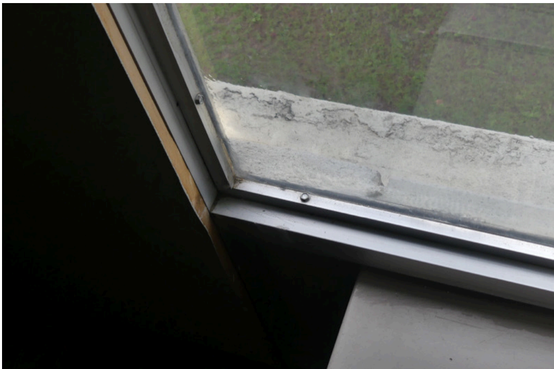
28. Guestroom 324, One Queen, Evidence of Moisture Intrusion at Window
