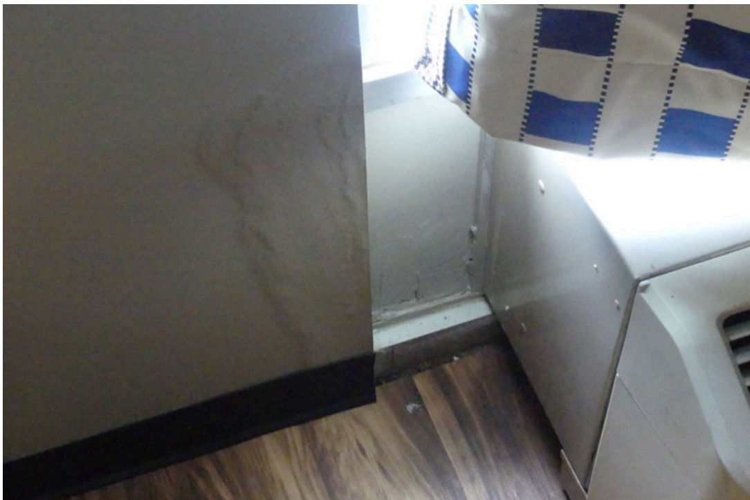
30. Guestroom 337, One Queen, Evidence of Past Moisture Penetration Adjacent to PTAC
