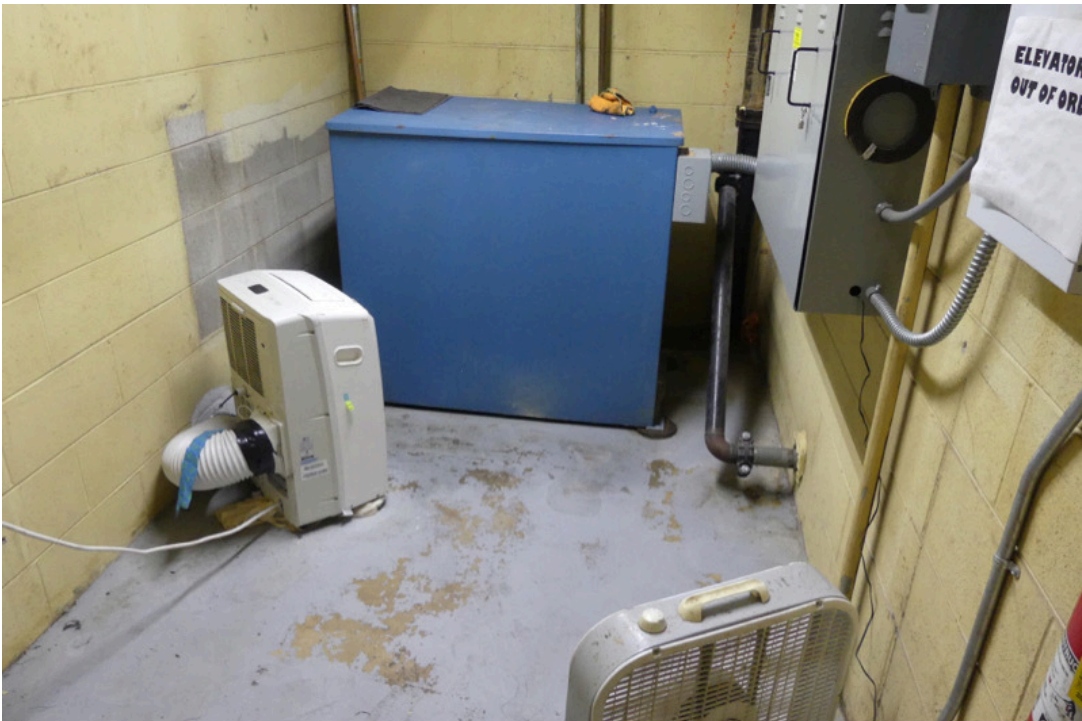
20. Hydraulic elevator equipment
