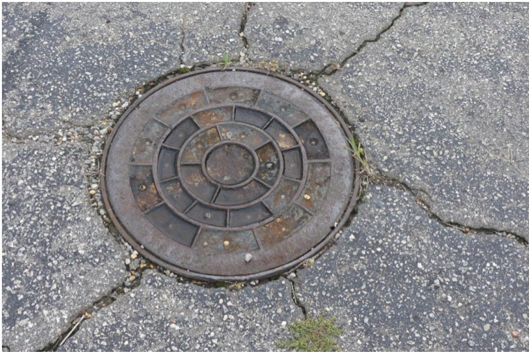
13. Grease trap access port
