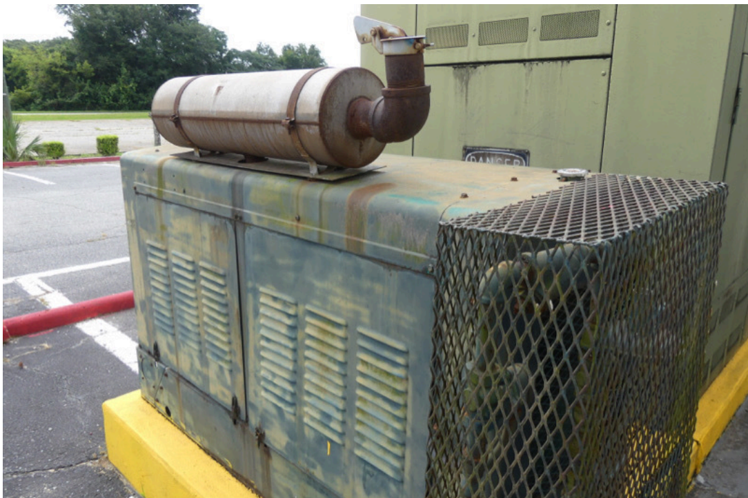
14. Out-of-service emergency generator
