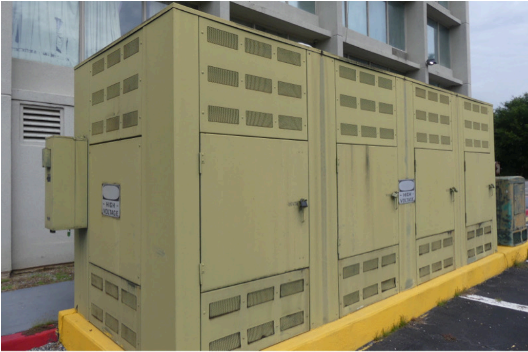
15. Pad-mounted transformer
