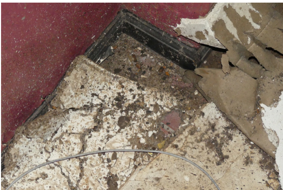
48. Damaged friable ACM in the former restaurant space
