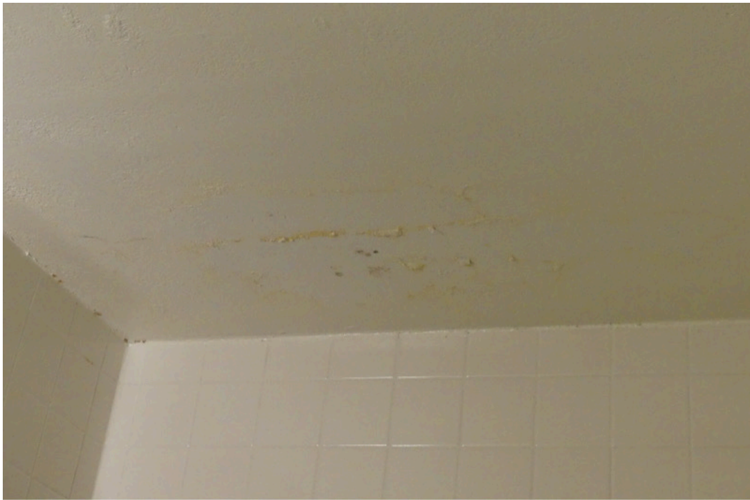
29. Guestroom 334, One Queen, Bathroom, Evidence of Past Condensation, Paint Failure
