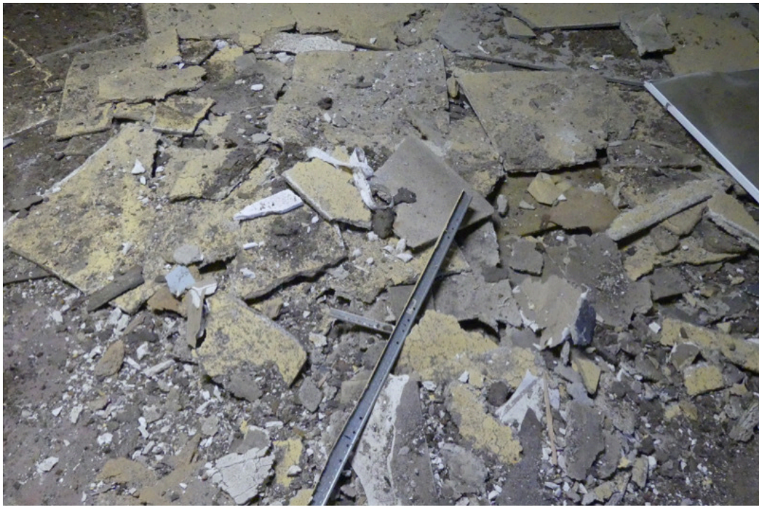
49. Damaged friable ACM in the former restaurant space
