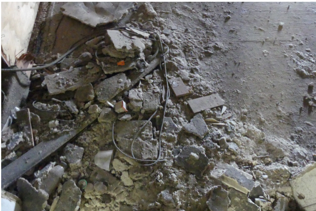
50. Damaged friable ACM in the former restaurant space
