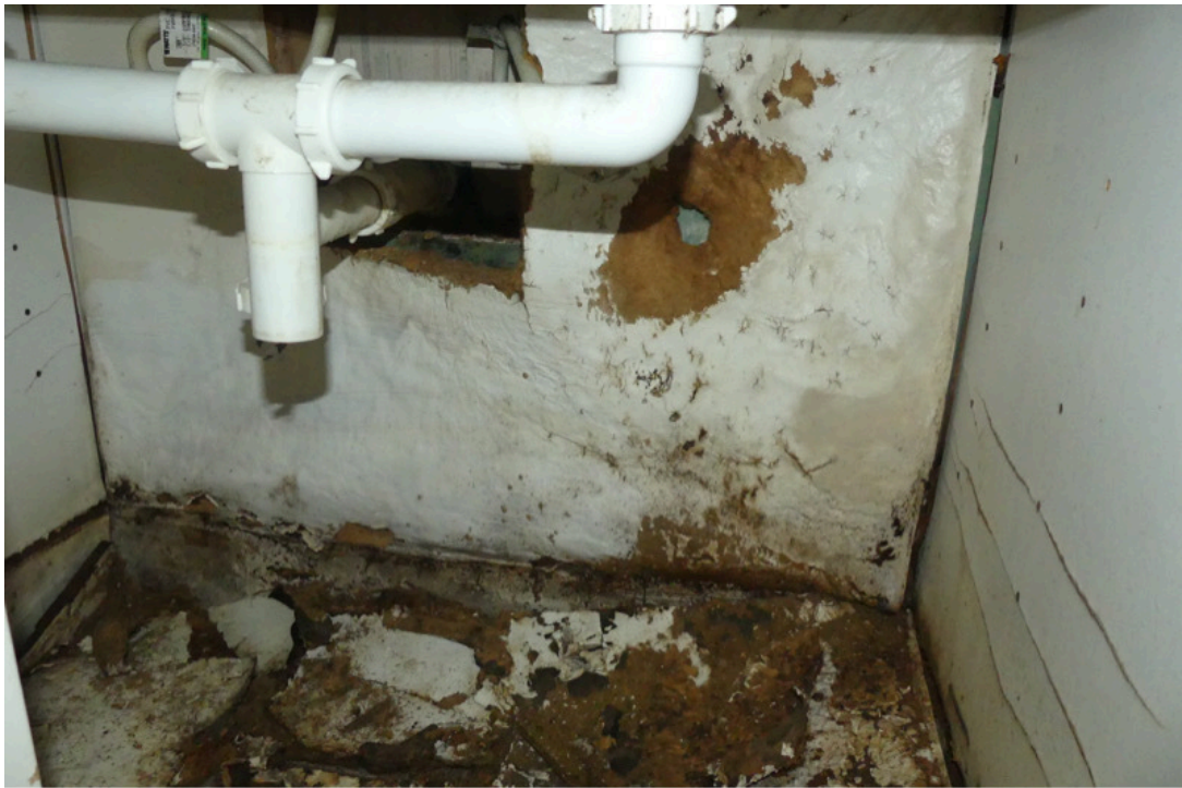
33. Guestroom 240, Manager's Apartment, Bathroom 2, Under Sink, Disconnected Drain and Water Damage
