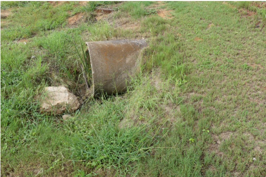
10. Concrete culvert
