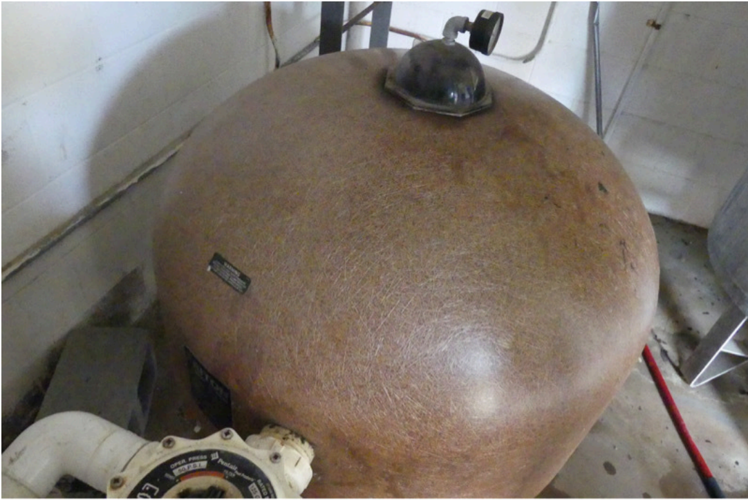
19. Pool equipment room filter
