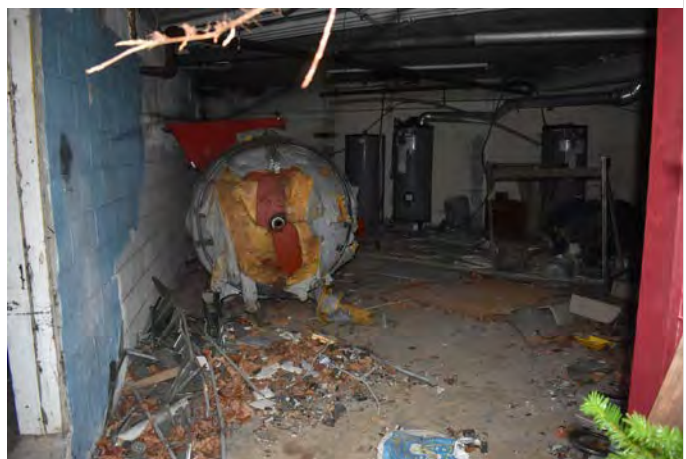
12. Suspect asbestos insulation on old water boiler
