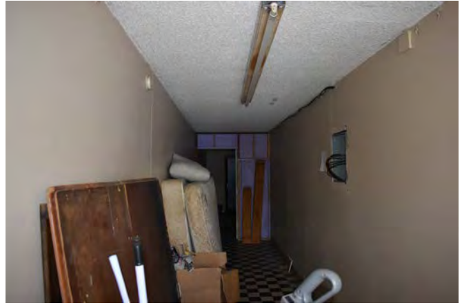
20. Interior maintenance corridor Building 1
