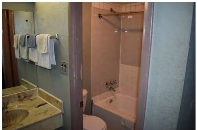
24. Interior typical room Building 2
