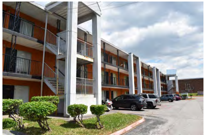
4. South side Building 1
