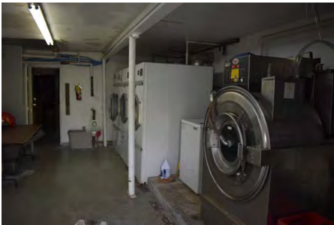
21. Interior laundry room Building 1
