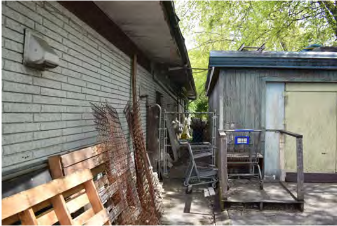
13. South side restaurant building
