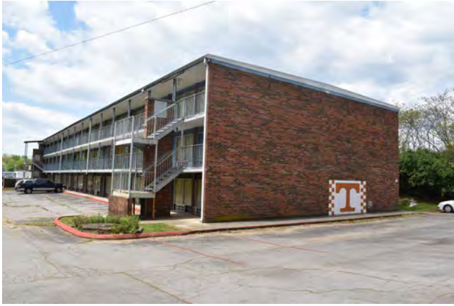
7. South and east sides Building 2
