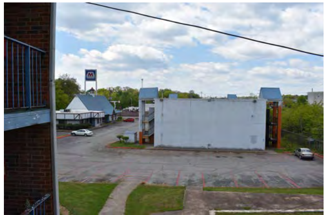
6. East side Building 1
