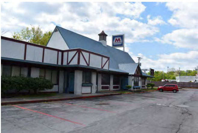
11. North side restaurant building
