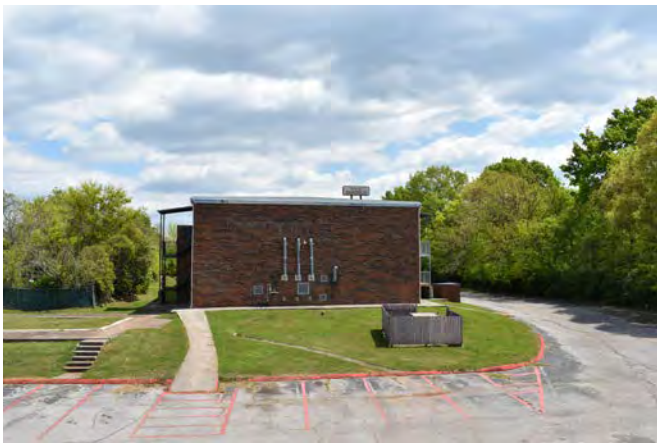
9. West side Building 2
