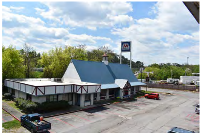
10. Roof and north and east side restaurant building
