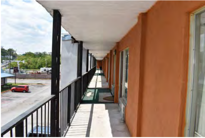
19. Typical exterior corridor Building 1
