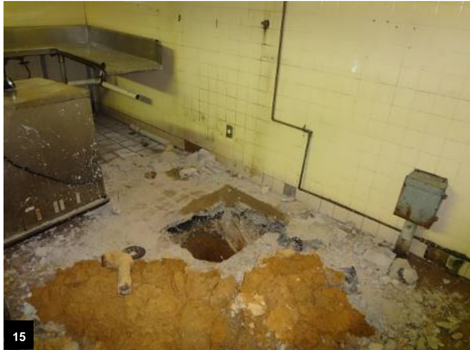
Plumbing replacement project in kitchen
