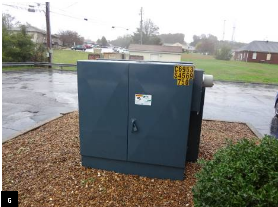
Utility-owned, pad-mounted transformer
