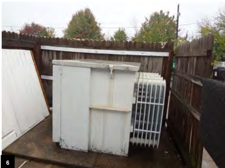
Utility-owned, pad-mounted transformer
