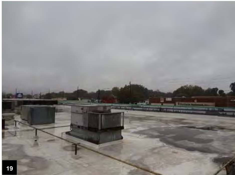
View of Subject's roof and HVAC package units
