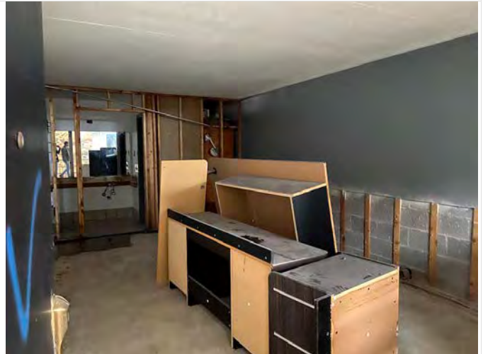
16. Room under construction
