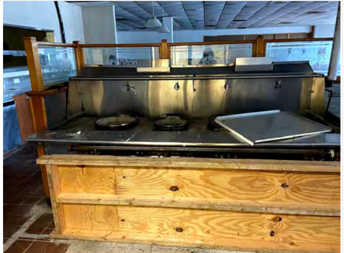
10. Restaurant (under construction)
