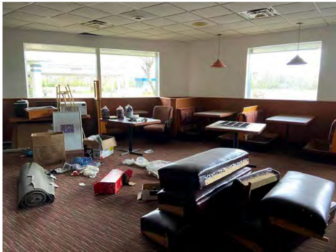
11. Restaurant (under construction)
