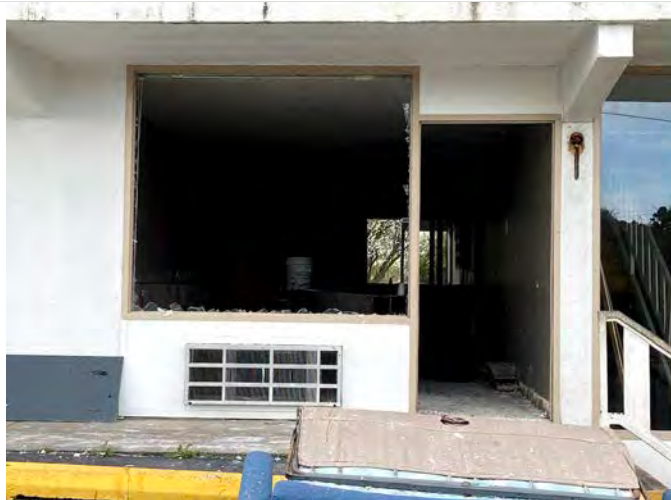
15. Room under construction
