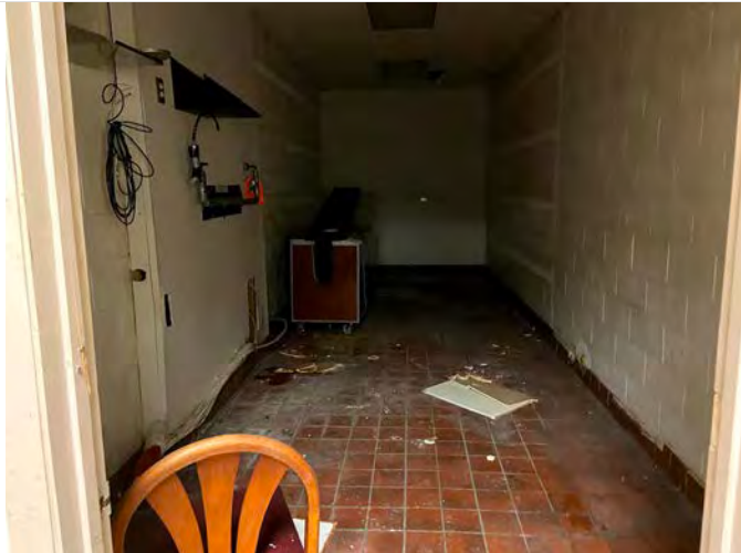
9. Restaurant (under construction)
