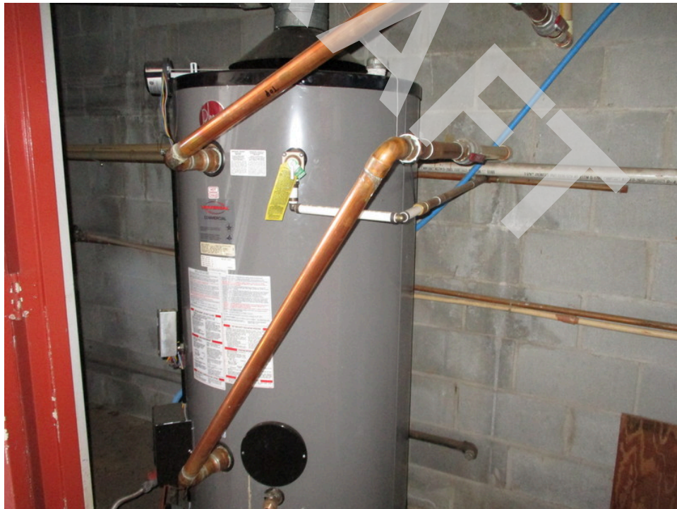
32. Typical gas fired water heater in 1006 Saint Patricks Drive
