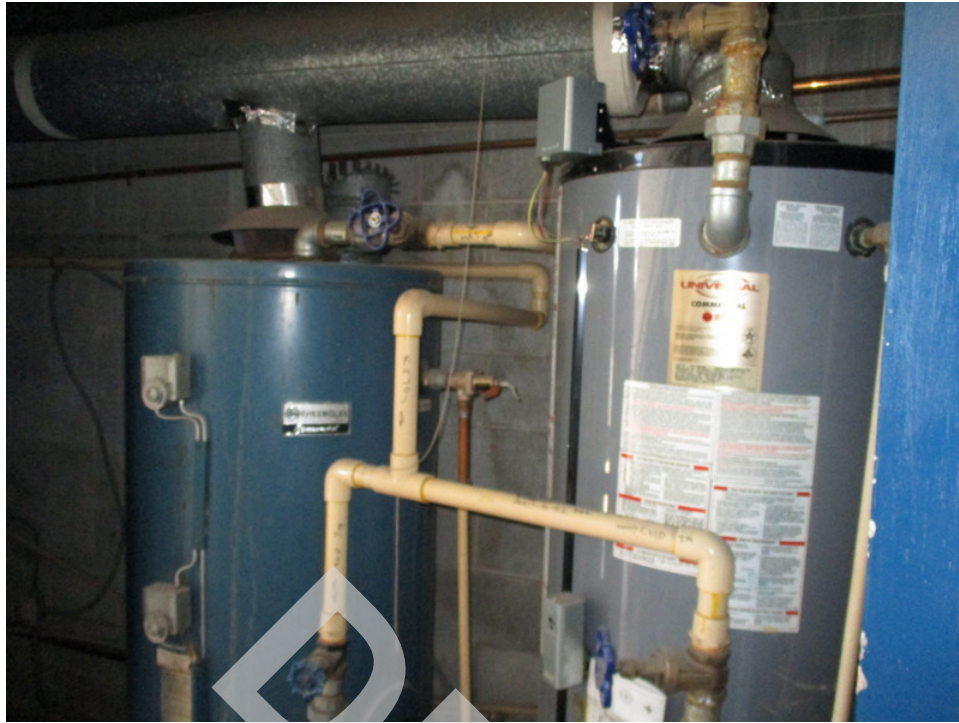
21. Typical gas fired water heaters in 1004A Saint Patricks Drive
